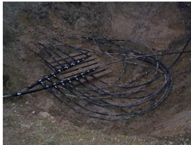
Underground manifold connections
