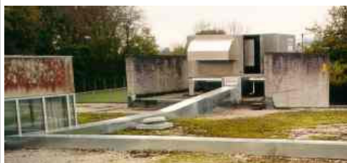
Ducted air system
