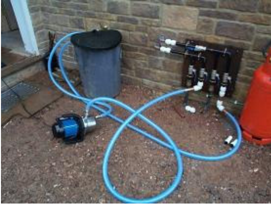
Purging an installed slinky system.
