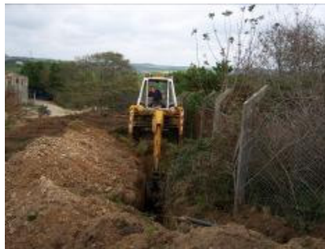
Slinky trench excavation
