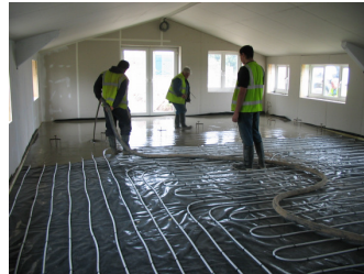
Screeding an underfloor system
