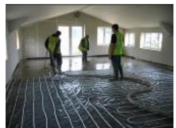
Screeding an underfloor system
