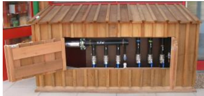
Fig 7 Header manifold connections
