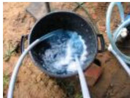
Fig 15 Purging the arrays of air
