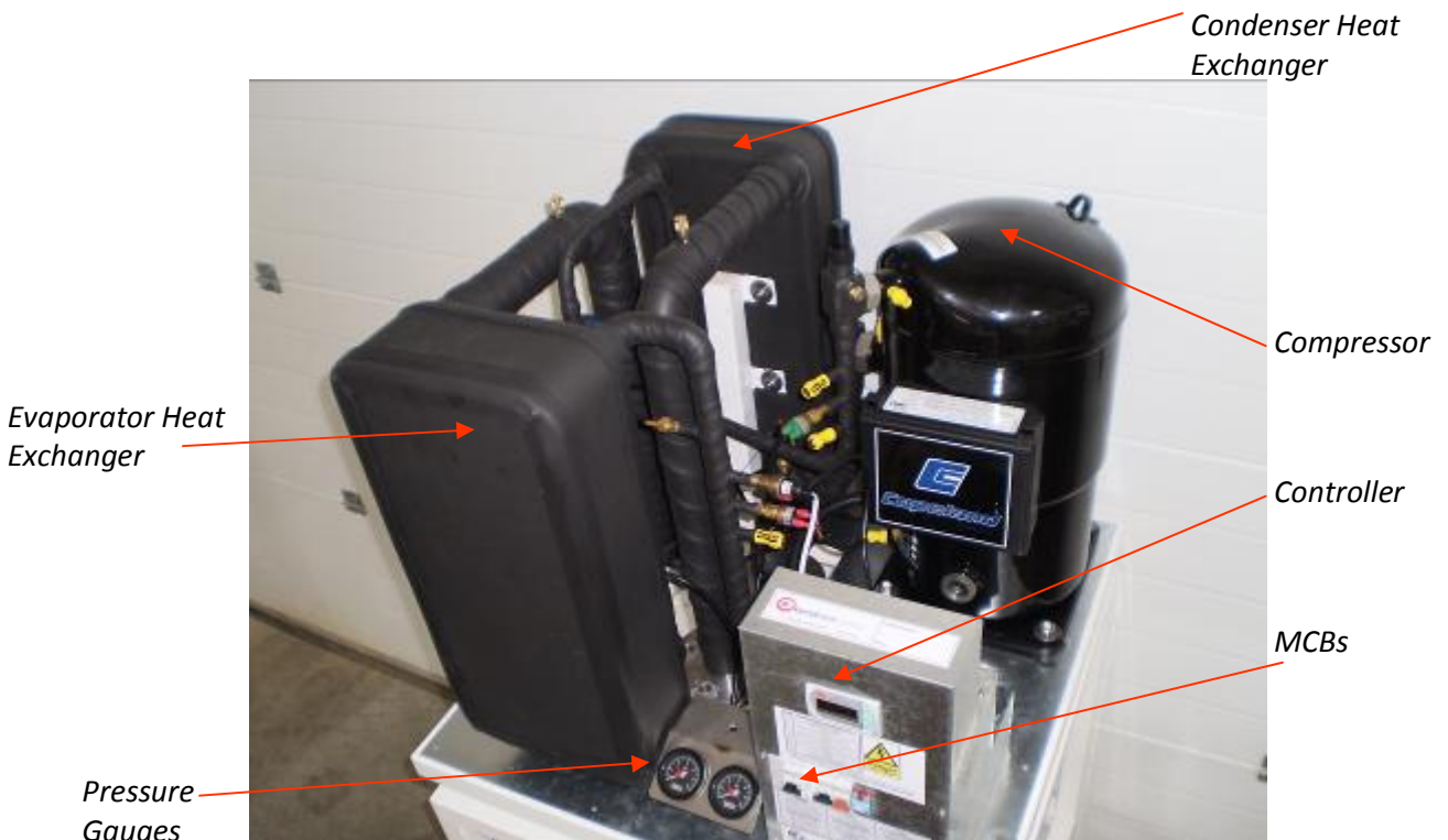
Fig 1. The internals of a heat pump
