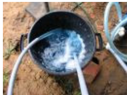
Fig 15 Purging the arrays of air
