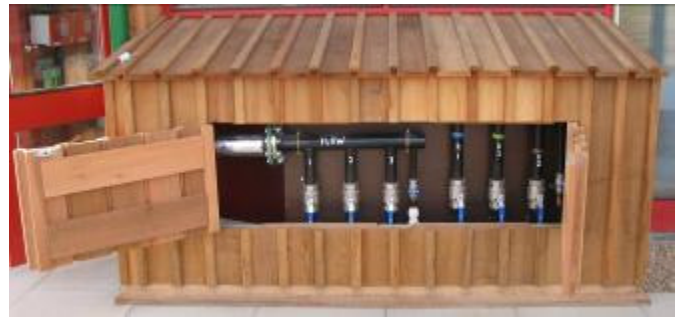
Fig 7 Header manifold connections
